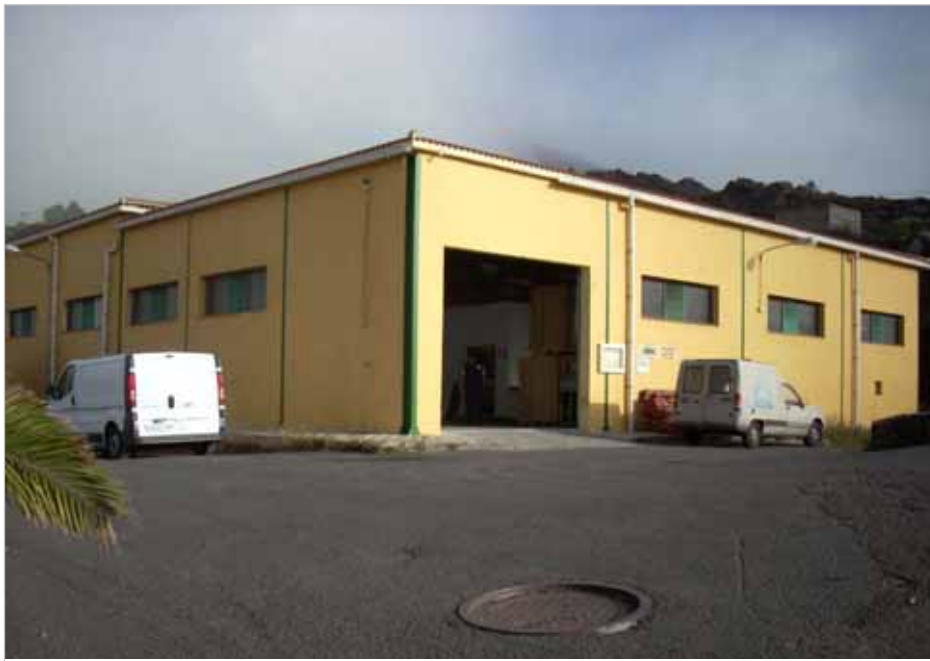
Warehouse for distributing Mercahierro S.A.U. products and administrative centre of the organisation
