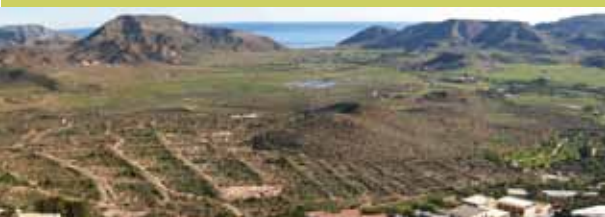
The Rodalquilar Valley. Here we can see an area of old mining spoil tips, now restored, and part of the Reserve's installations.
